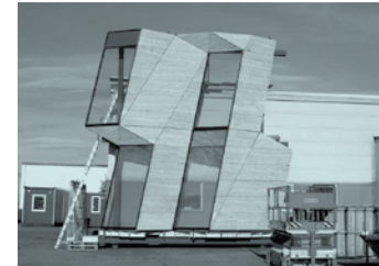
THE HORTEN BUILDING'S FAÇADE NOT ONLY SHADES THE INTERIOR FROM THE SUN BUT ALSO PROVIDES THE STRUCTURE OF THE BUILDING.
