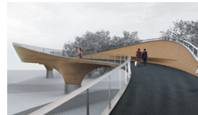
A gradient of less than 4 per cent offers users a gentle climb.
