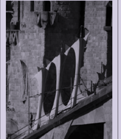
DEVELOPMENT OF THE COLONNADE DESIGN ABOVE THE NARTHEX (PASSION FAÇADE). THE COLUMNS HERE ARE PAINTED POLYSTYRENE PROTOTYPES MACHINED DIRECTLY FROM A 3D DIGITAL MODEL.
