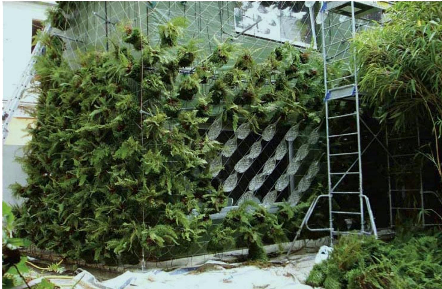
R&SIE(N) USED PARAMETRIC MODELLING ON THE FERN FAÇADE TO CONTROL THE DIMENSIONS AND THE TOPOLOGY OF THE SURFACE.
